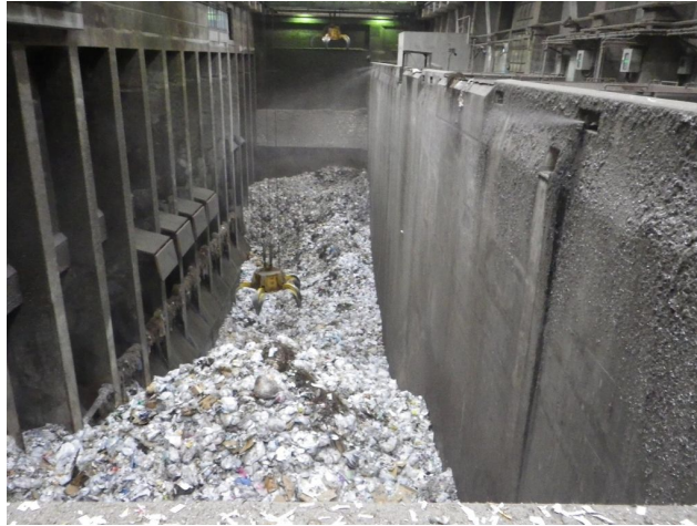
Shinagawa Incineration Plant
