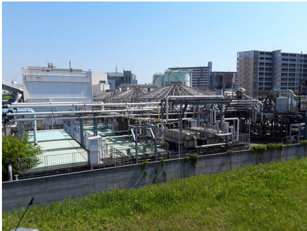
The Ebie Sewage Treatment Plant
